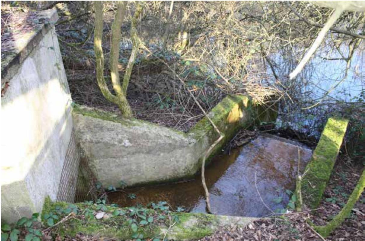
Rectangular outfall tank fed by a sluice shown on the revised edition OS map of 1976 labelled "Tank"; and on the 1994 masterplan of RAF Greenham as an "Outfall Tank" (RAF Greenham Common Masterplan Sheet 5 of 7). This is likely to be part of the airbase stormwater drainage system installed during the 1951 to 1953 reconstruction of the airbase.
