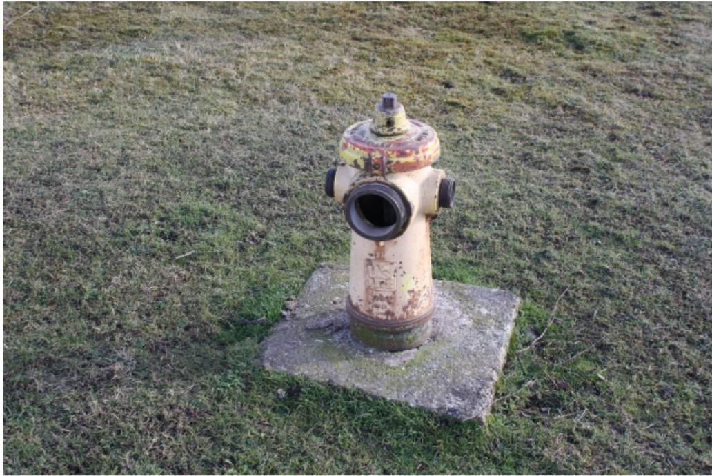
Iron fire hydrant with two side and one front cap, painted cream with brown top and side caps, with traces of red and yellow paint on the top and yellow paint on caps; standing to a height of 0.7 metres and set on a square concrete pad (c. 0.6 metres across). Has "VSP OPEN 5 1/4 VO" on the top; "655510 5 1/4 VO 10106 D1" on north side; "D1 US PIPE 1986 AWWA PAT. 4.123.285" on south side; and "TOPSIDE USP 668860" on south side base.
