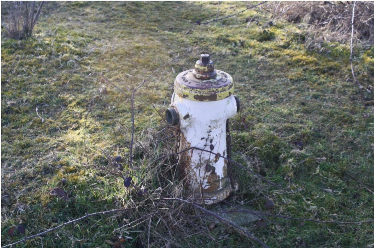
Iron fire hydrant painted cream with brown paint on the top and side caps, which also have traces of yellow paint (the front side cap is missing); standing to a height of 0.7 metres and set on a square concrete pad (c. 0.6 metres across). Has "VSP OPEN 5 1/4 VO" on the top; "655510 5 1/4 VO 10106 D1" on one side; "D1 US PIPE 1986 AWWA PAT. 4.123.285" on the other side above "TOPSIDE USP 668860" on the base.
