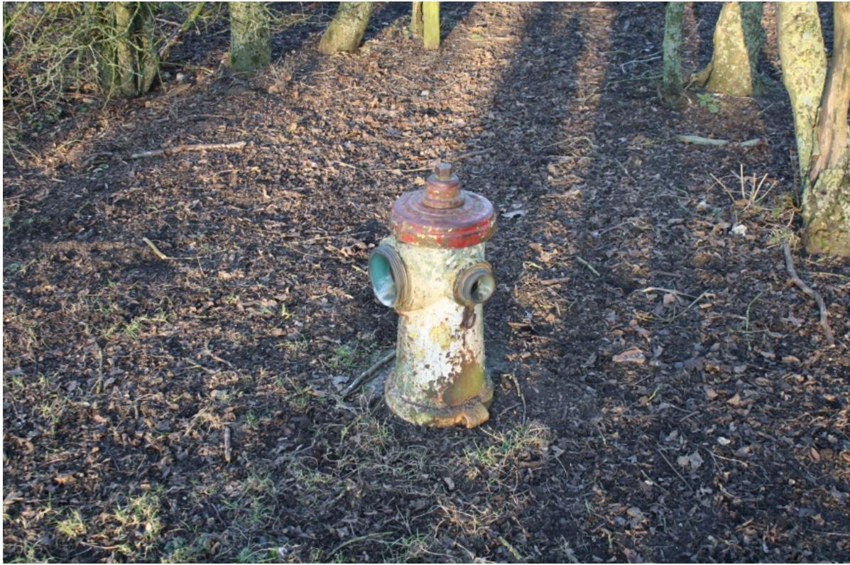
Iron fire hydrant painted cream with brown, red and yellow paint on the top, which also has traces of yellow paint (all three of the side caps are missing); standing to a height of 0.7 metres and set on a square concrete pad (c. 0.6 metres across). Has "VSP OPEN 5 1/4 VO" on the top; "655510 5 1/4 VO 10106 D1" on one side; "D1 US PIPE 1986 AWWA PAT. 4.123.285" on the other side above "TOPSIDE USP 668860" on the base.
