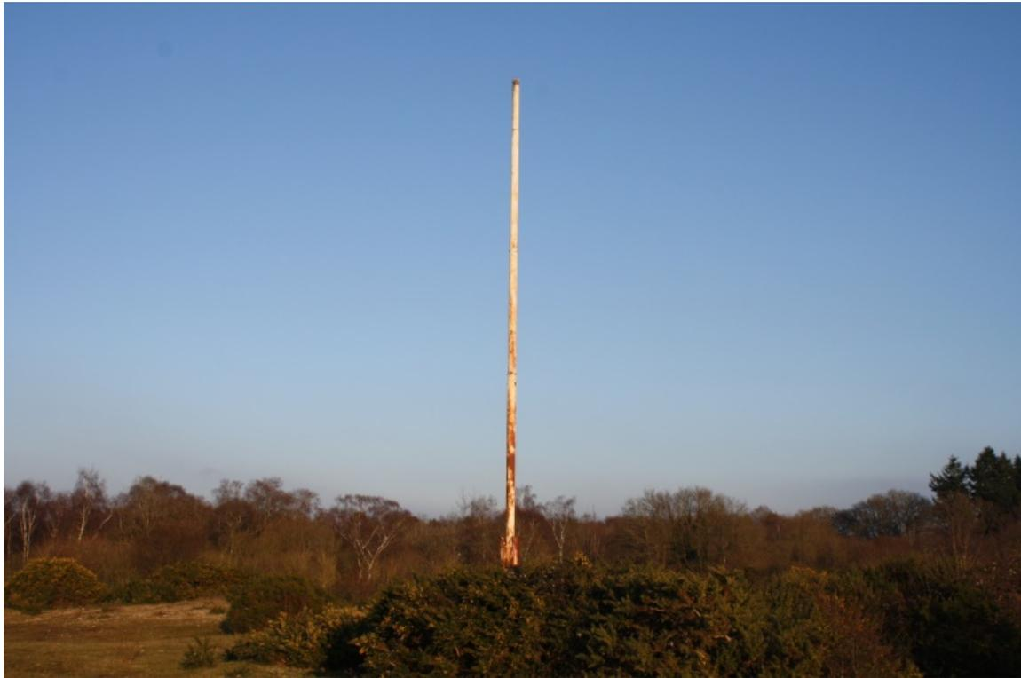
Flag pole made from three tubular sections secured by a bolt to two I beams with large weights at one end near the base (for lowering the pole). The pole is set in a square concrete slab (1.5 metres across). The I beams are stamped "B.S.C. GLENGARNOCK G.T. BRITAIN". Produced by the British Steel Corporation in the Glencarnock works which were taken over from Colvilles in 1967 and closed in 1985 (Grace's Guide Glencarnock Iron and Steel Company).
