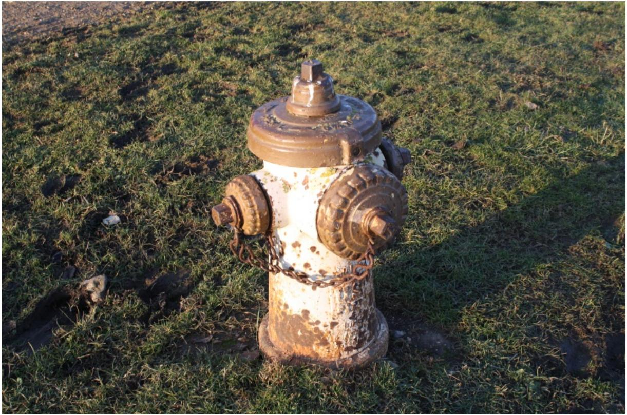
Iron fire hydrant painted cream with brown paint on the base, top and side caps, which also have traces of yellow paint; standing to a height of 0.7 metres and set on a square concrete pad (c. 0.6 metres across). Has "VSP OPEN 5 1/4 VO" on the top; "655510 5 1/4 VO 10106 D1" on one side; "D1 US PIPE 1986 AWWA PAT. 4.123.285" on the other side above "TOPSIDE USP 668860" on the base.
