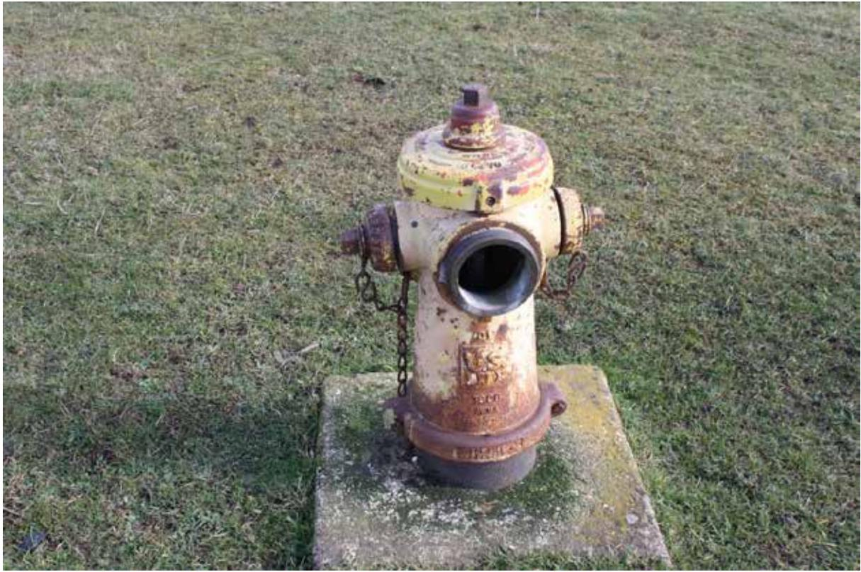
Iron fire hydrant painted cream with brown paint on the top and side caps, which have traces of red paint and have a yellow top coat (the front cap is missing); standing to a height of 0.7 metres and set on a square concrete pad (c. 0.6 metres across). Has "VSP OPEN 5 1/4 VO" on the top; "655510 5 1/4 VO 10106 D1" on one side; "D1 US PIPE 1986 AWWA PAT. 4.123.285" on the other side above "TOPSIDE USP 668860" on the base.
