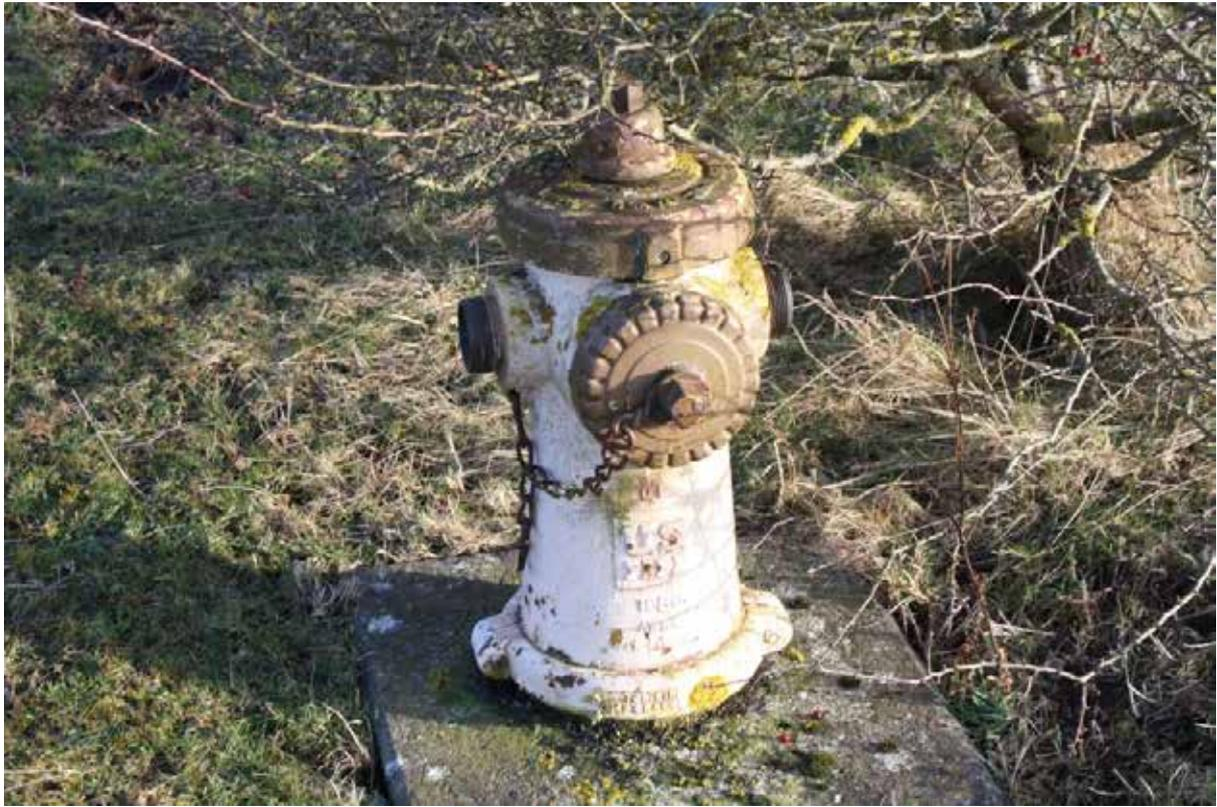
Iron fire hydrant painted cream with brown paint on the top and front cap, which also have traces of yellow paint (the side caps are missing) standing to a height of 0.7 metres and set on a square concrete pad (c. 0.6 metres across). Has "VSP OPEN 5 1/4 VO" on the top; "655510 5 1/4 VO 10106 D1" on one side; "D1 US PIPE 1986 AWWA PAT. 4.123.285" on the other side above "TOPSIDE USP 668860" on the base.
