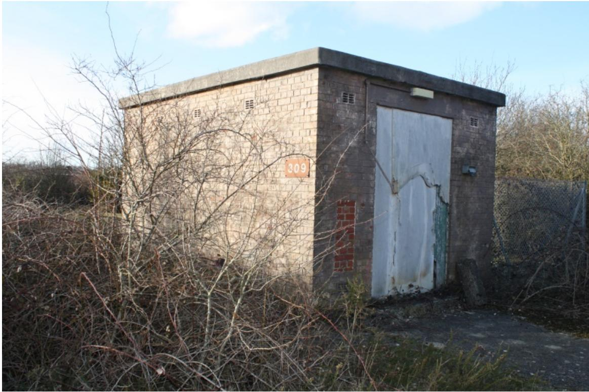
Small electricity sub-station constructed with modern brick (marked with military building number plaque 309) with a broken plank constructed wooden door on the eastern side and a wire and mesh compound to the north. The approach road and part of its kerb is still visible. Can be seen on the 1975 record site plan (Greenham: A Common Inheritance Website); the 1994 masterplan of RAF Greenham (RAF Greenham Common Masterplan Sheet 2 of 7); and an AP taken 16th May 1998.
