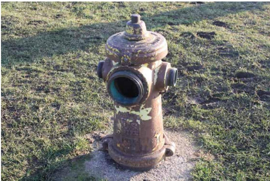
Iron fire hydrant with traces of cream and yellow paint (all three of the side caps are missing); standing to a height of 0.7 metres and set on a square concrete pad (c. 0.6 metres across). Has "VSP OPEN 5 1/4 VO" on the top; "655510 5 1/4 VO 10106 D1" on one side; "D1 US PIPE 1986 AWWA PAT. 4.123.285" on the other side above "TOPSIDE USP 668860" on the base.
